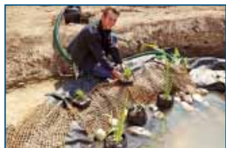
7. Planting on level areas Lay out coconut mats for planting level areas. They provide an optimal opportunity for plants to take root.
