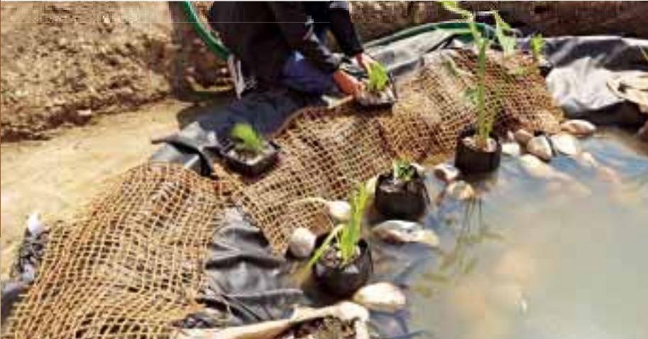
Application example: Embankment mat
